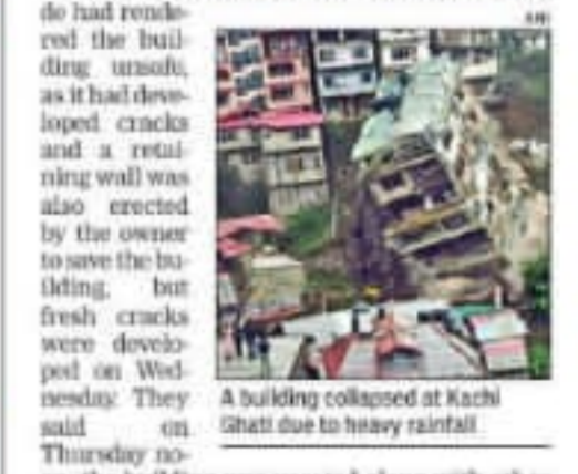
A building collapsed at Kachi Ghati due to heavy rainfall.
